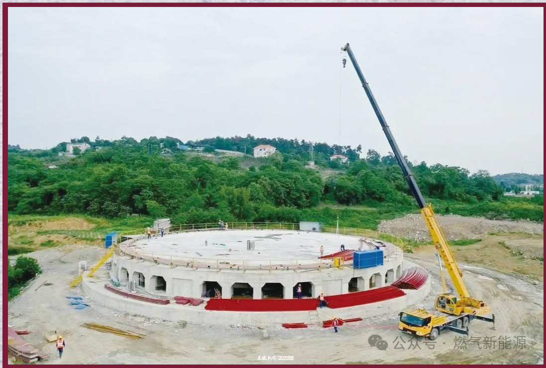
遵义天然气液化调峰储备站储罐基础
